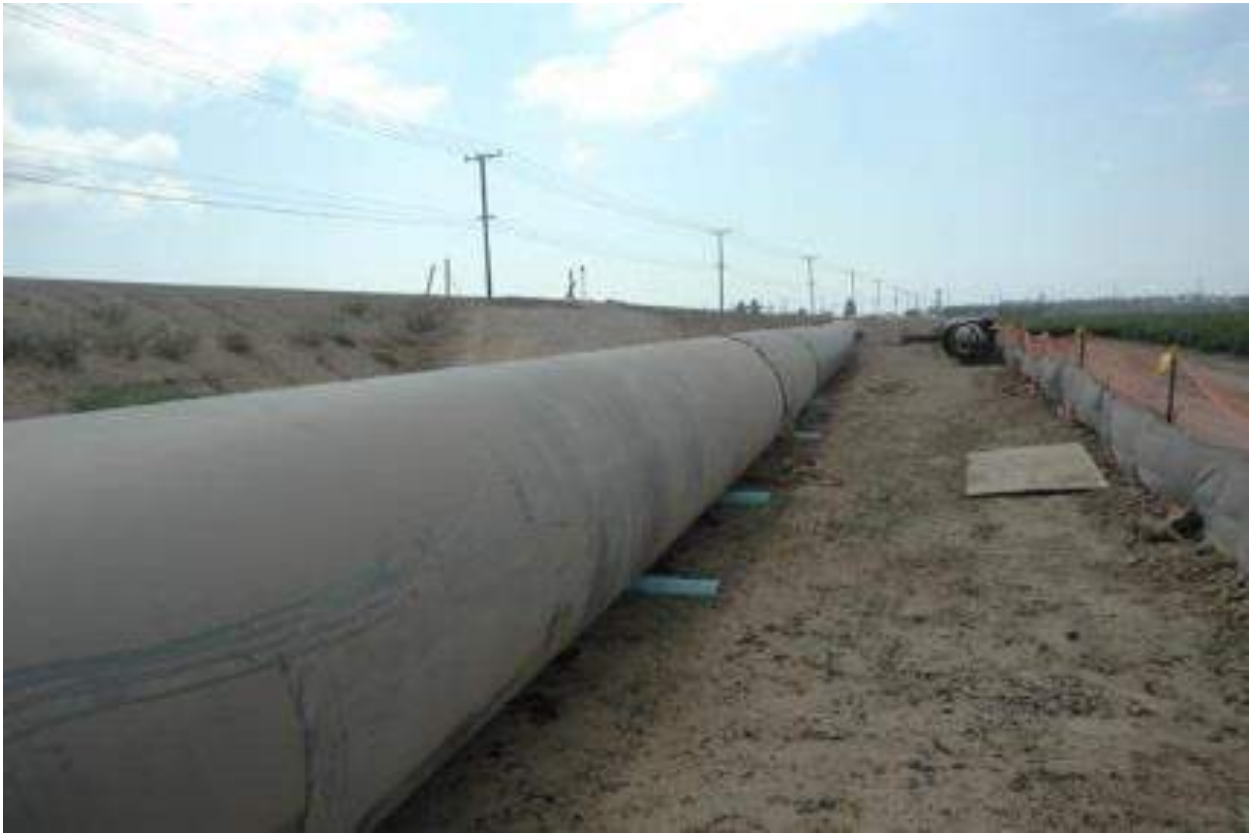
Fig. 26 The Calleguas salinity management pipeline, in Ventura County, California, under construction in 2007.
